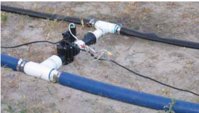
Figure 11. Solenoid valves connected to a timer allow sequential irrigation of different zones. Credits: Eric Simonne.
