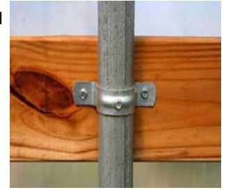
Figure 16: Fastening batten board to frame.
