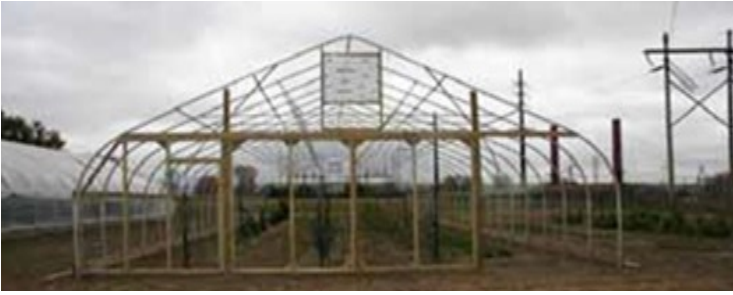
Figure 18: Peak-style (gothic arch) high tunnel framing—front view showing end wall framing. Large doors open outwards at both end.
