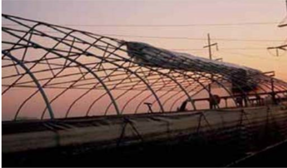
Figure 25: Applying the plastic over the high tunnel superstructure.
