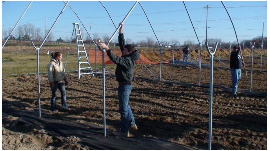
Figure 23: Multi-bay hoops are installed on ground posts (legs).
