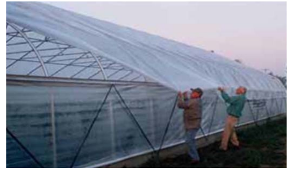
Figure 27: Fastening plastic to hipboards.
