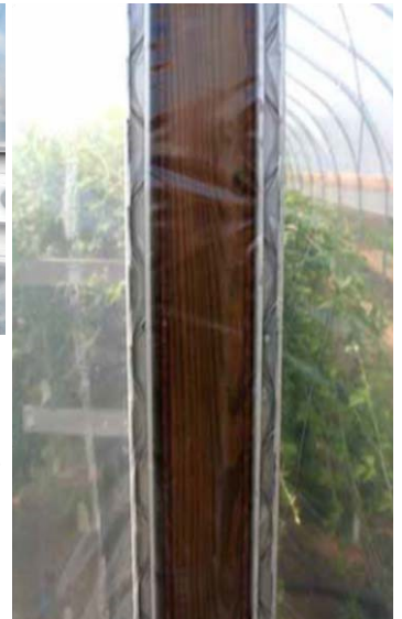
Figure 31: Plastic film attached to the end wall of a tunnel with aluminum extrusions (attached to the wooden frame) and zig-zag wire (wiggly wire). The zig-zag wire secures the film by holding it in place inside the aluminum (U-shaped) extrusion. The zig-zag wire can be easily removed when the plastic needs to be replaced. While the zig-zag wire can be used multiple times, it is often replaced when new plastic is installed.
