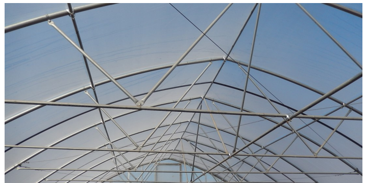
Figure 14: Wider tunnel with more structural support.
