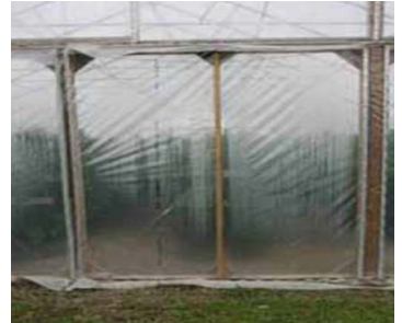
Figure 19: Door covered in plastic.
