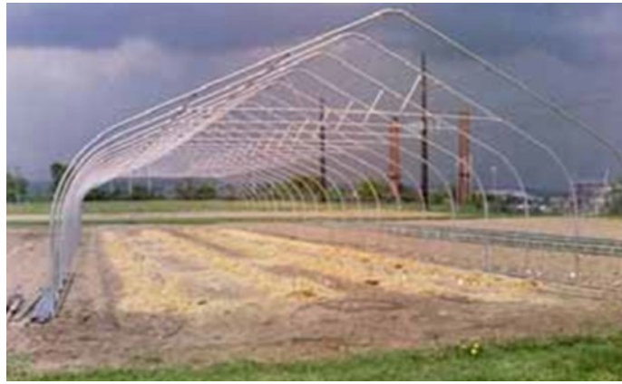
Figure 7: Peak-style (gothic arch) high tunnel during construction and prior to the installation of the plastic film cover, Ithaca, NY.
