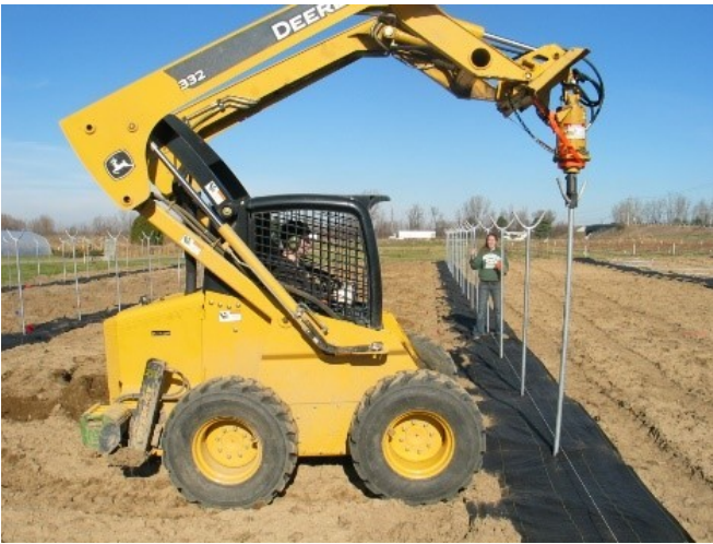
Figure 22: Multi-bay tunnels; ground posts (legs) are augered in at pre-marked positions.
