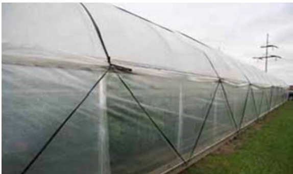
Figure 28: Webbing applied over plastic to keep it from blowing in the wind.
